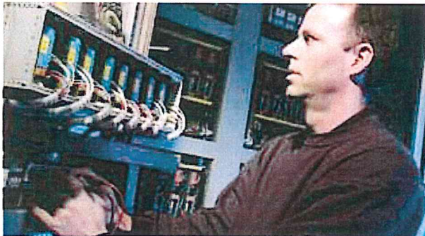
Inspection & auditing to optimize system settings including software modification.
